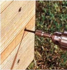
TimberLok deck install...
