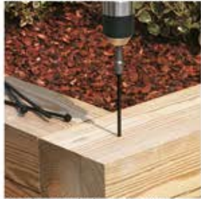
TimberLok beams insta...
